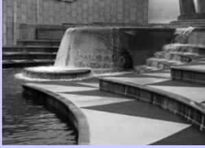
Lake Lenexa Dam Photo by Kim Feldkamp Dam Safety Team Leader
