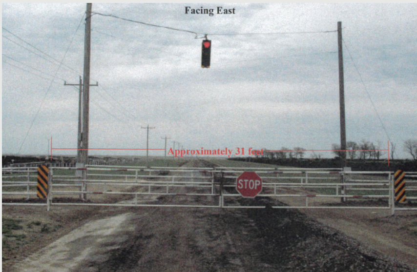
FIGURE 5. Gate at feed lot to move cattle across the road. Object markers are fine but STOP sign should be replaced with road closed sign. Note blinking light, which is helpful to warn traffic, but not an MUTCD requirement.
