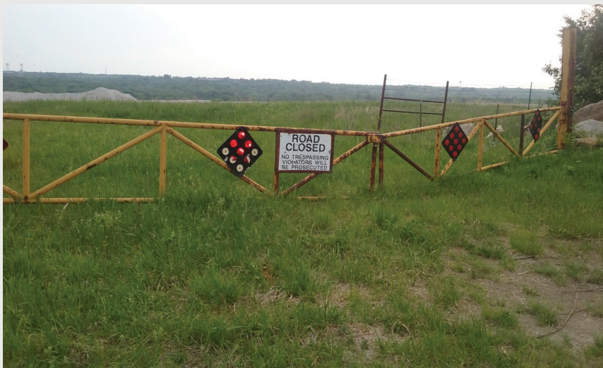
FIGURE 6. It is easy to overlook maintenance of gates and related signing.
