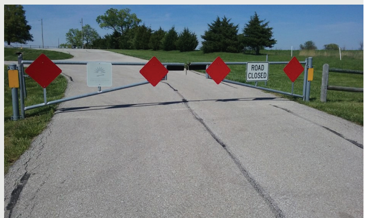
FIGURE 2. Proper way to sign a gate with ROAD CLOSED sign, OM-4 end of road markers, and object markers on gate posts.
